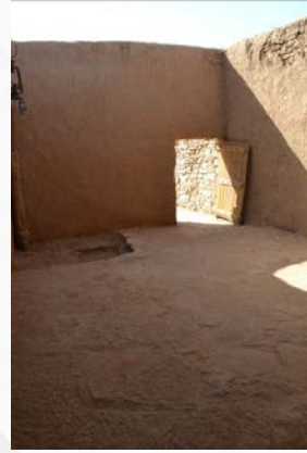
b. Males's entrance leading to visitors' courtyard
