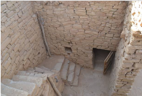
c. Staircase from the courtyard to upper floor
