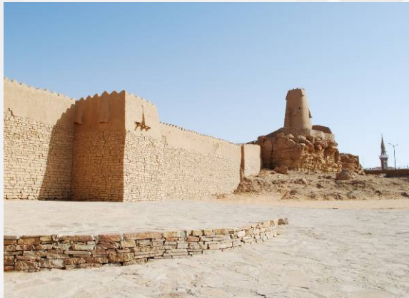
Fig. 6 The castle's western fence where the entrance is located (Source: Author)
